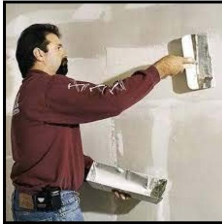
**Figure 3 – Example of Applying Wet Joint Compound**
