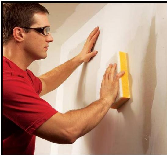
Figure. 5 – Example of Wet Sanding
