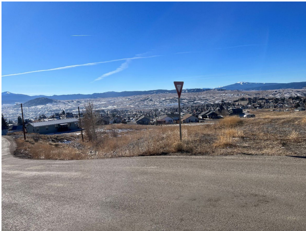
Photograph 4. Maintenance road access and rock lined channel on the east side of site.
