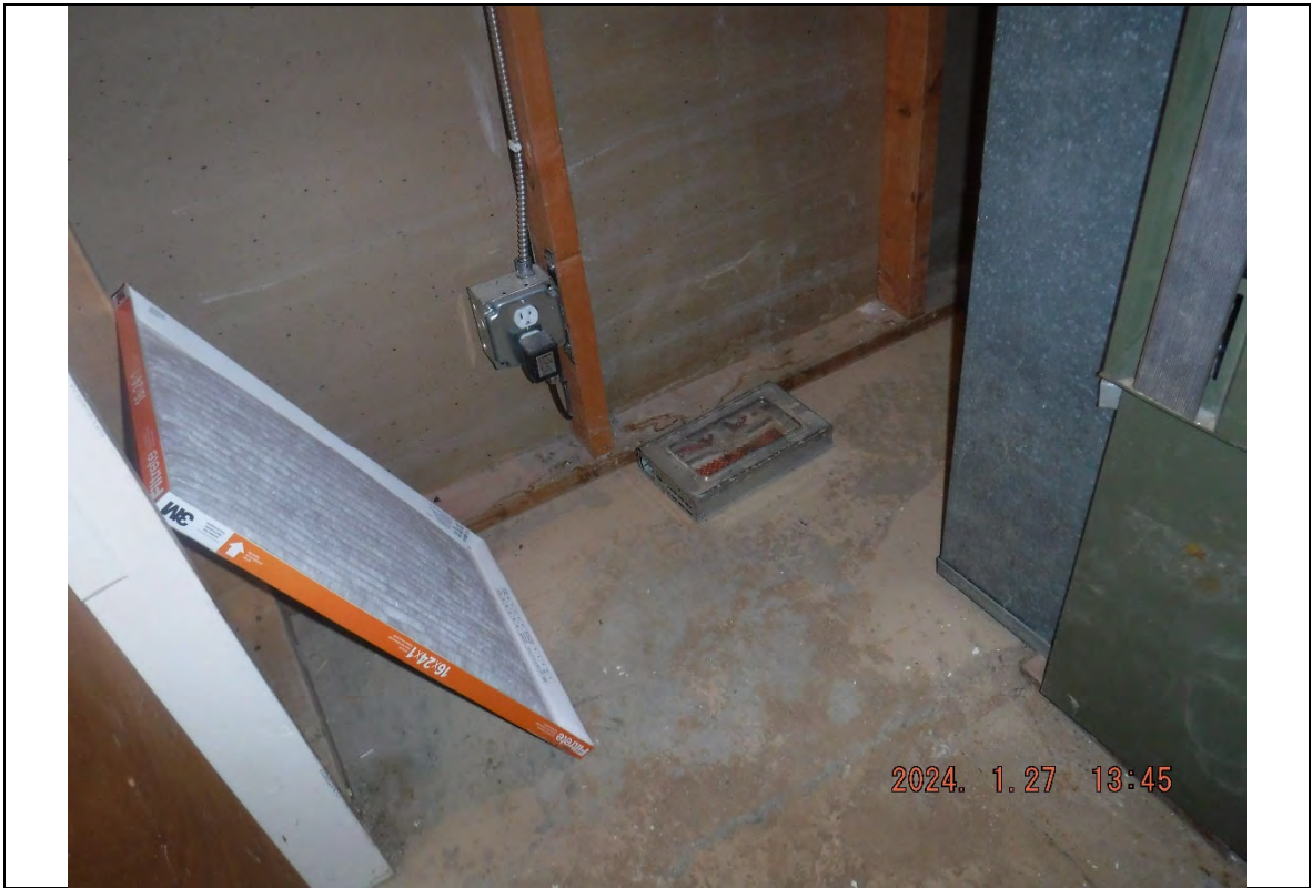
Photograph: 2235 Furnace room floor, facing southeast.
