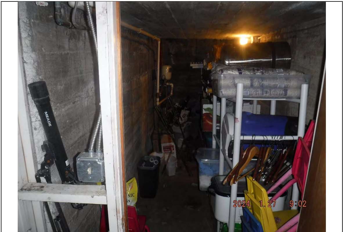
Photograph: 2221 North storage closet, prior to cleaning, facing north.
