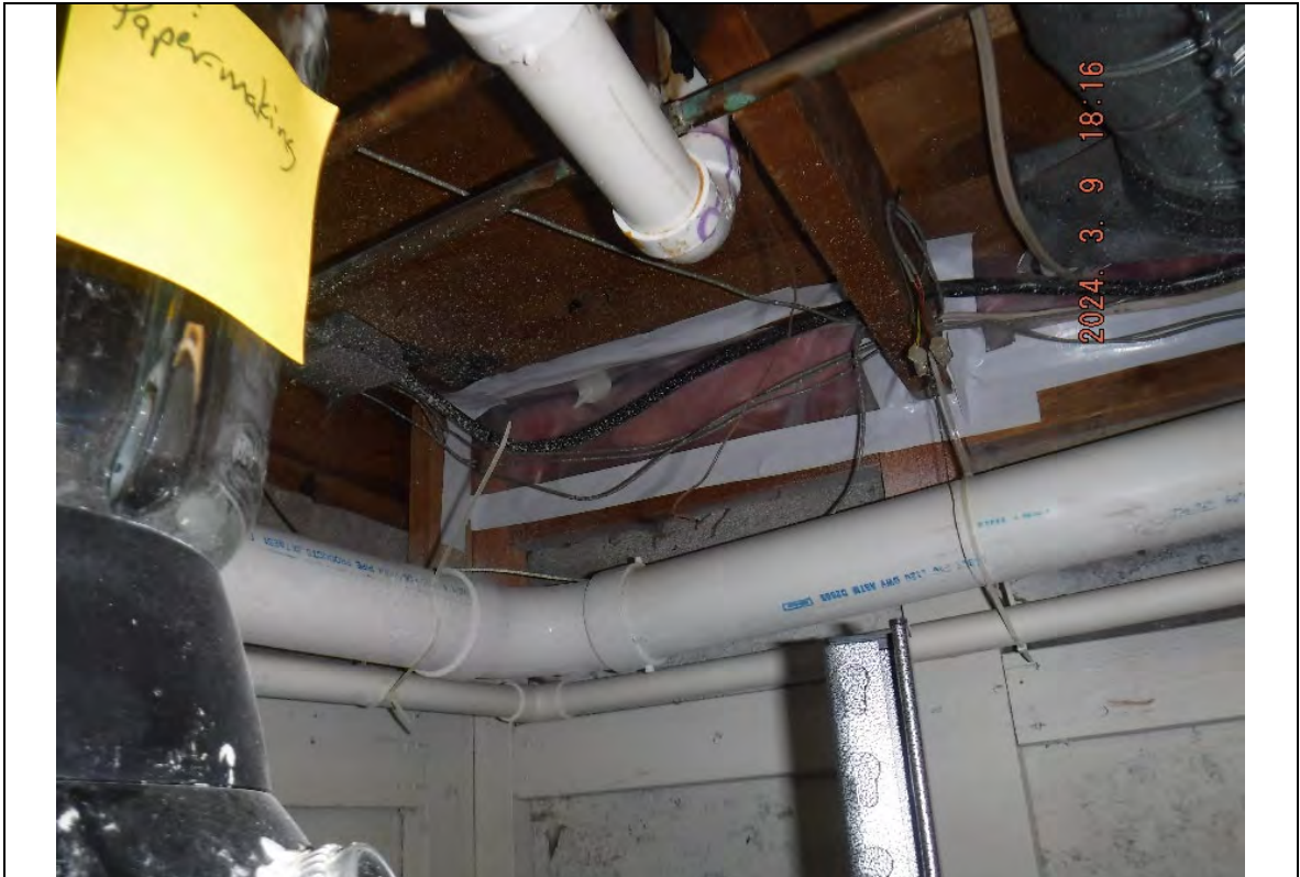
Photograph: 2444 Sealed insulation, northwest side of basement, facing northwest.
