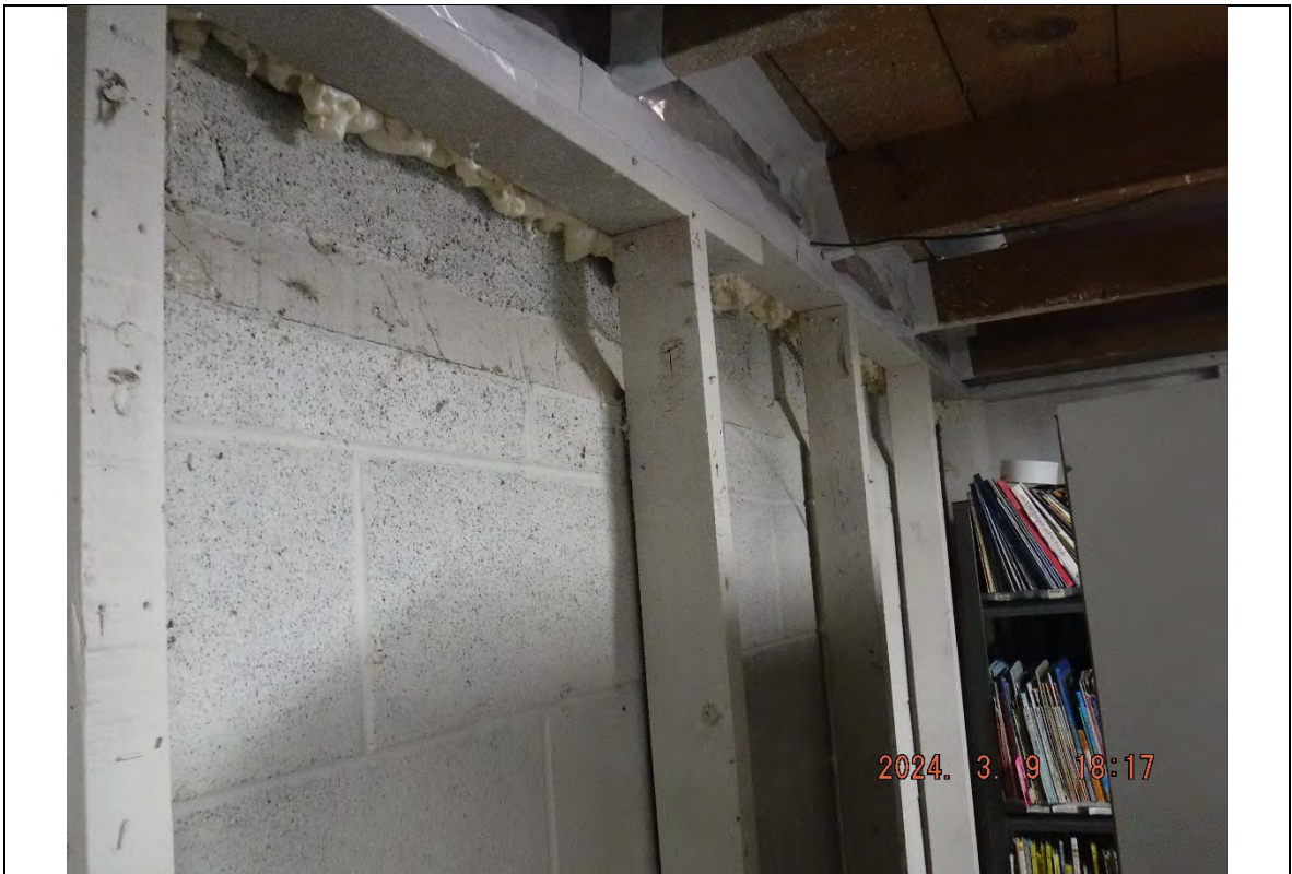
Photograph: 2248 Insulation foam, south side of basement, facing west.
