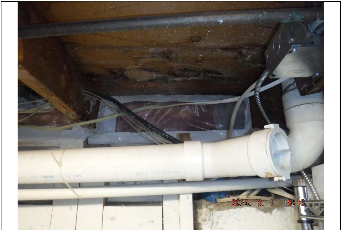
Photograph: 2445 Sealed insulation, north side of basement, facing north.
