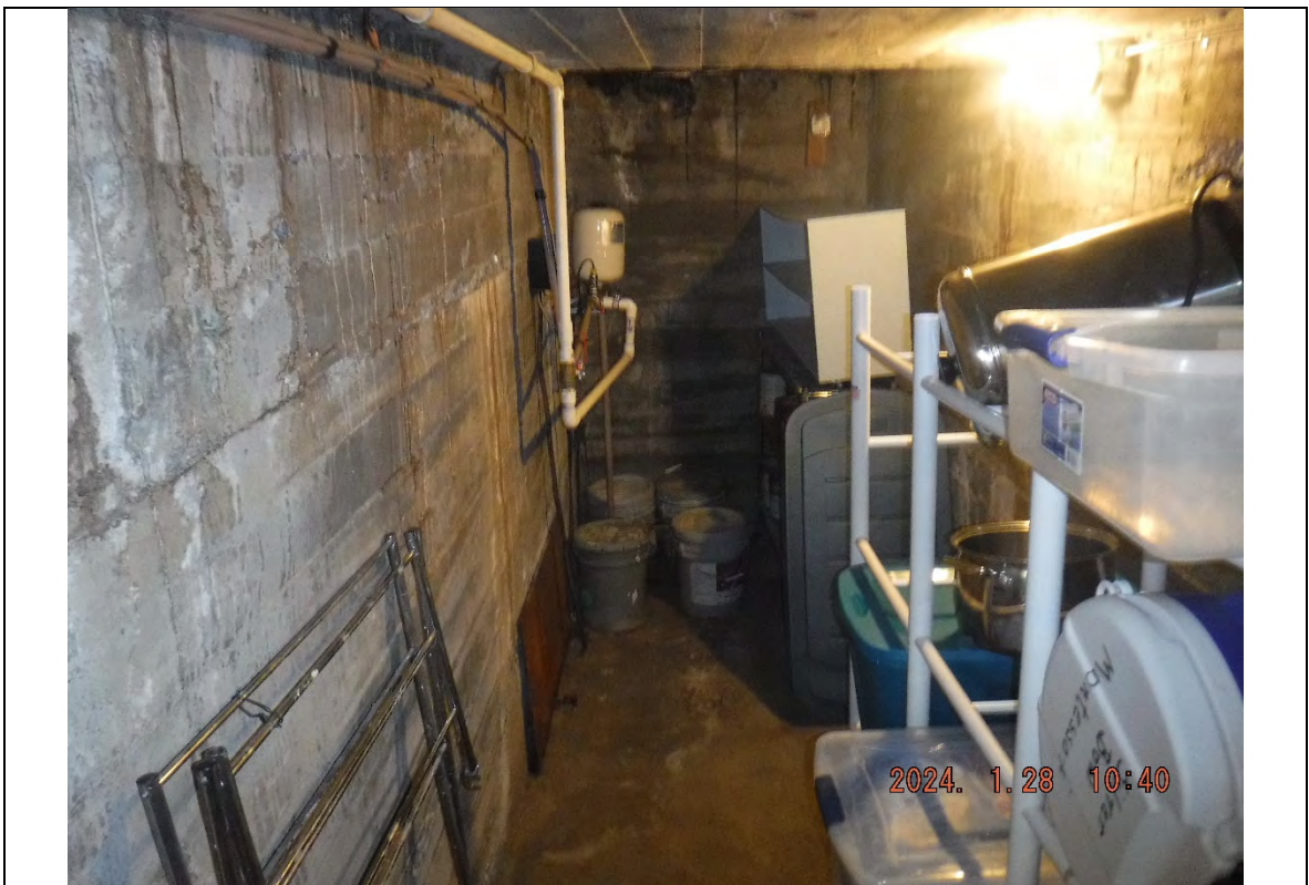
Photograph: 2255 North storage closet, following initial cleaning, facing north.
