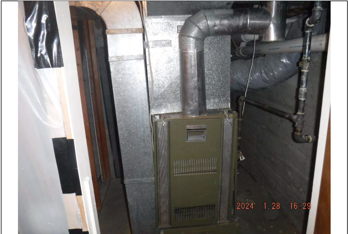
Photograph: 2271 Furnace room, following final cleaning, facing south.
