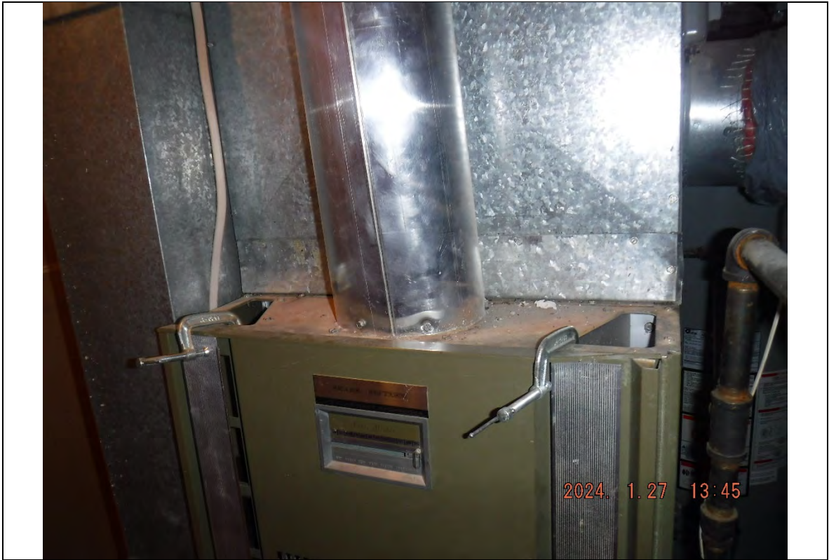
Photograph: 2234 Furnace room, top of furnace, facing south.
