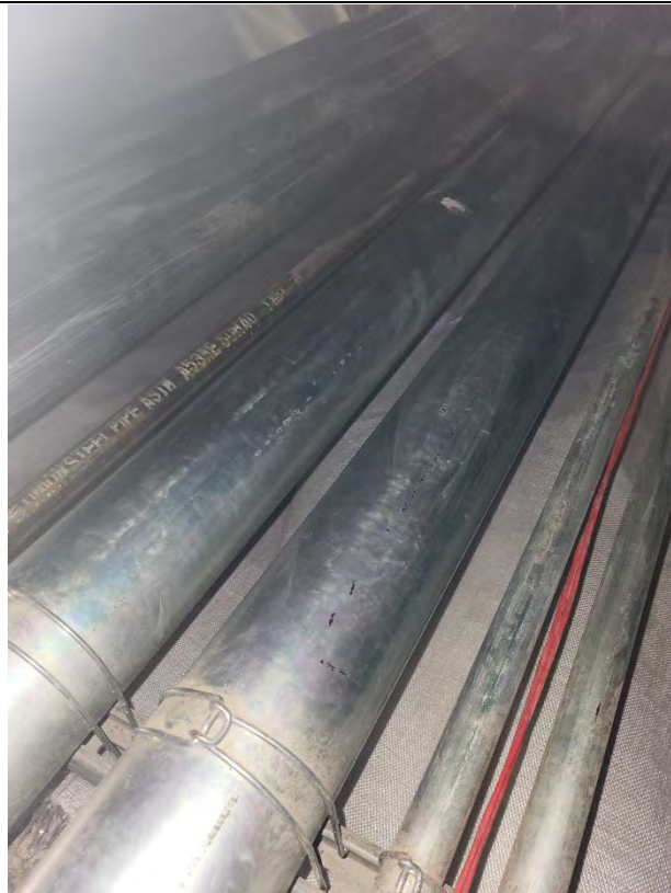
Photograph: 6 Pipes after they were wiped down, near the northern boiler room entrance. All horizontal surfaces in crawl space were wiped down with tri-phosphate wipes.
