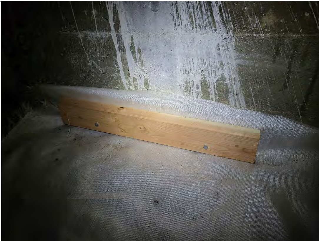
Photograph: 18 | The fabric could not be secured to the earthen crawl space with stakes or adhesive (soil material was too fine for stakes, adhesive would not stick to tarp material), so 2x4s were adhered to each corner of concrete walls, and additional 2x4s were drilled to the tarp and to the 2x4s adhered to the wall.
