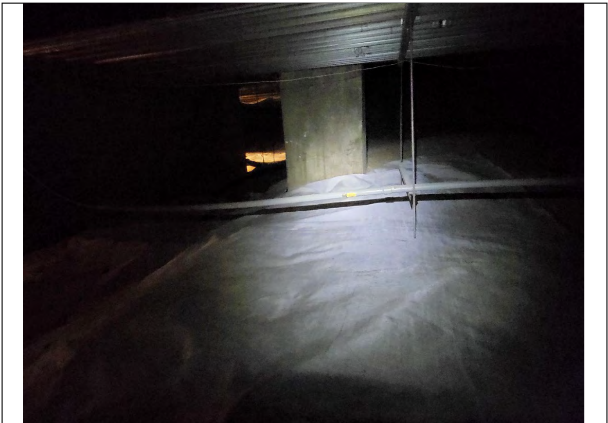
Photograph: 24 | South entrance of crawl space, with geo-textile fabric, facing west.
