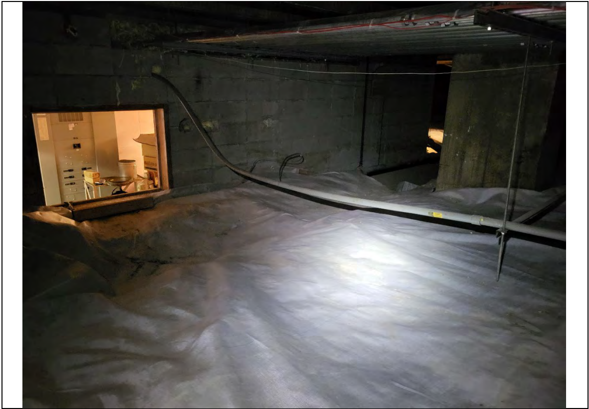
Photograph: 23 | South entrance of crawl space, with geo-textile fabric, facing southwest.
