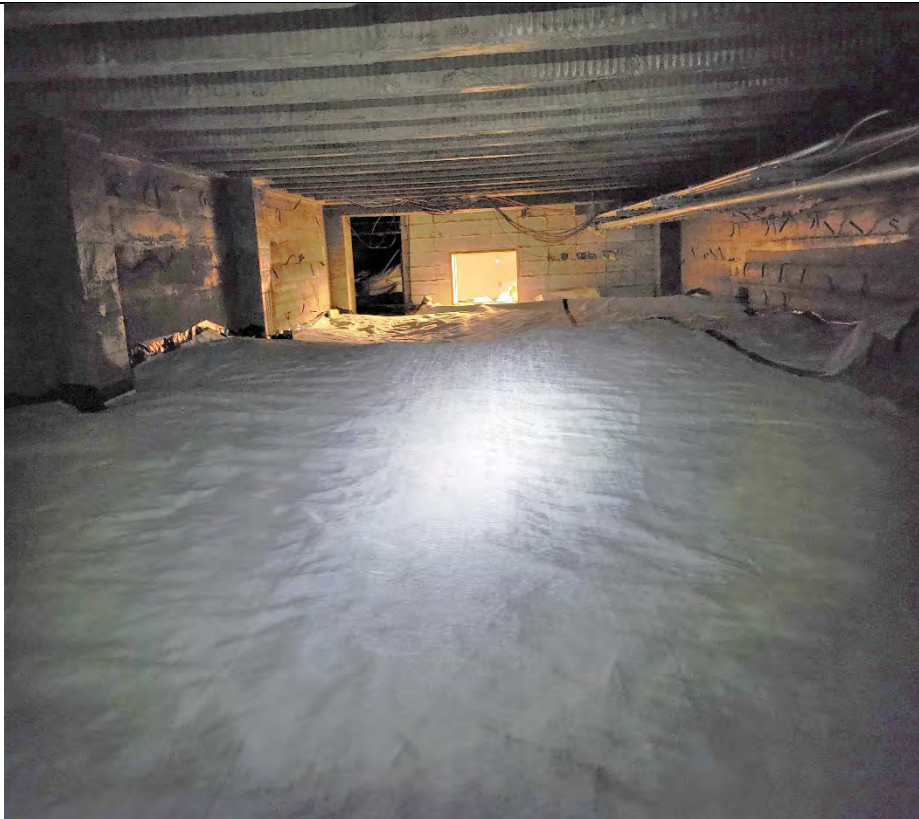
Photograph: 17 | Geo-textile fabric, fixed to southwest crawl space entrance, facing east.
