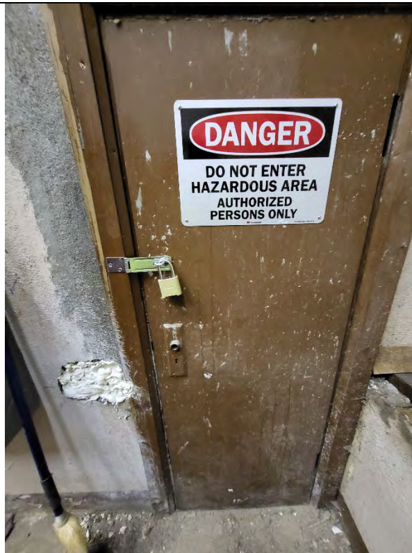
Photograph: 8 Door in boiler room with aluminum sign stating: "Danger: Do Not Enter Hazardous Area Authorized Personnel Only". Door would not close, so door hinges were removed to allow for door to be closed properly. A double hinge hasp was installed, and combination lock was used to lock the door. The combination was given to administrative staff.
