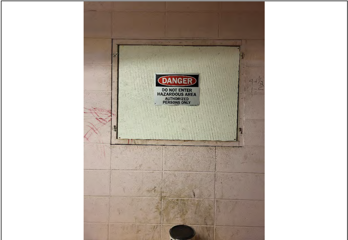
Photograph: 10 Southwest crawl space entrance, sealed with screws and attached aluminum sign stating "Danger: Do Not Enter Hazardous Area Authorized Personnel Only".
