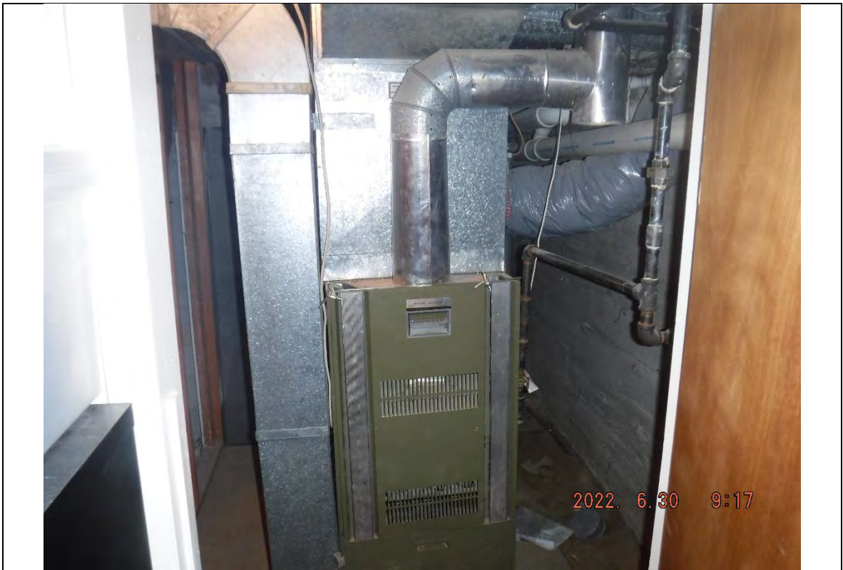
Photograph: Furnace/boiler room entrance, facing south. 0411
