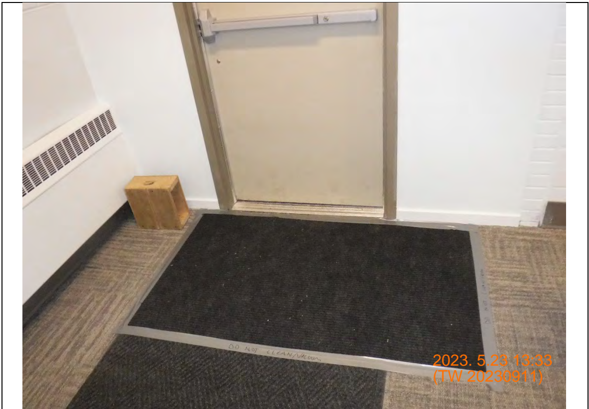
Photograph: 1684 Floor surface sample, east entrance by playground (S-0013-D-FM-03-20230523).
