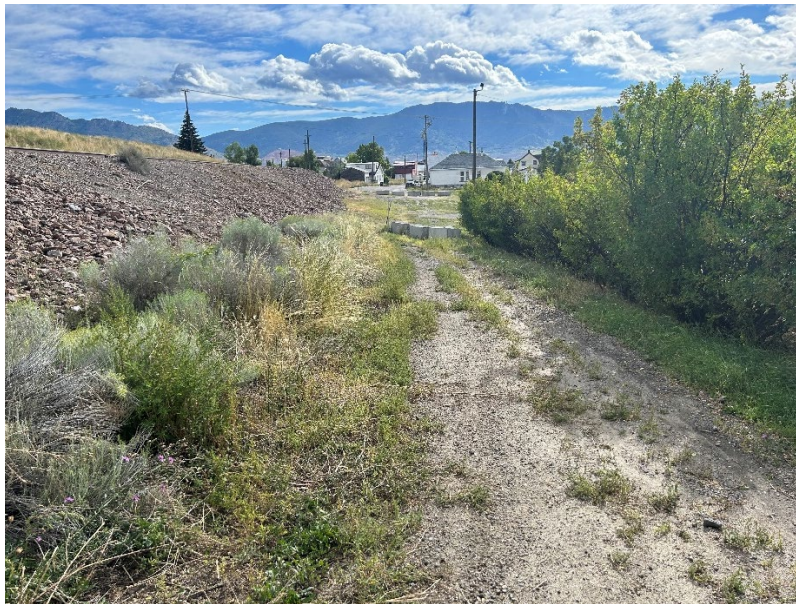
Photograph 4: Gravel road south of railway, facing east. Willows and ground cover prevent sediment and ground cover migration from road and railbed to the south.
