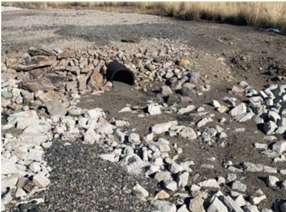
LY-D-01: Sediment accumulation and thin rock cover on the Southwest side.
