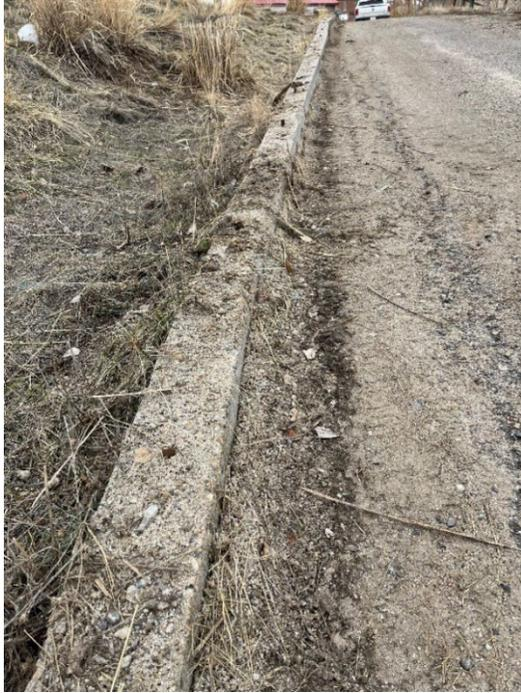
Photograph 3: Erosion and sediment on the east side of site facing north.
