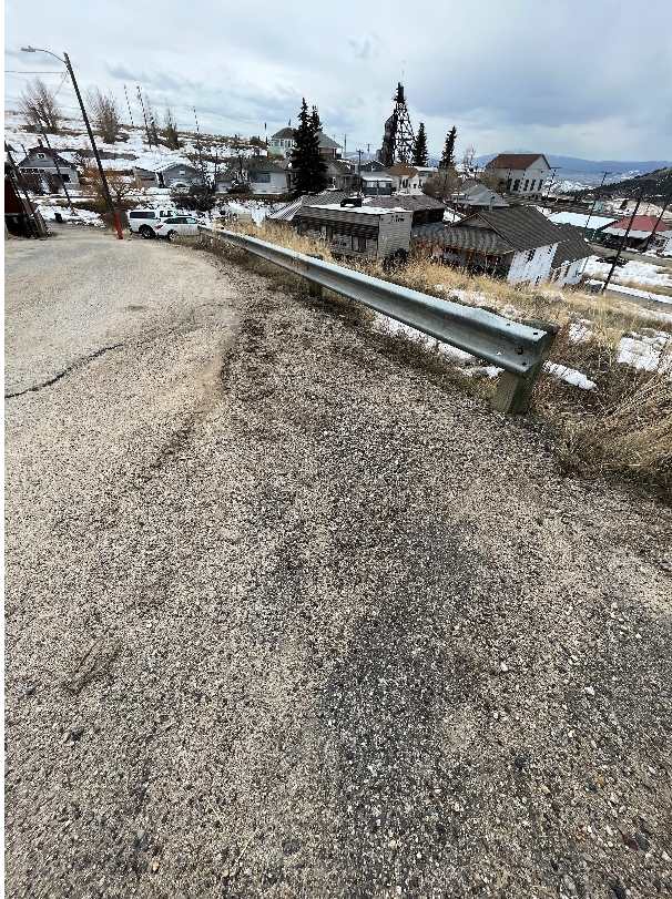
Photograph 3: Sediment from properties above Clayton Street.
