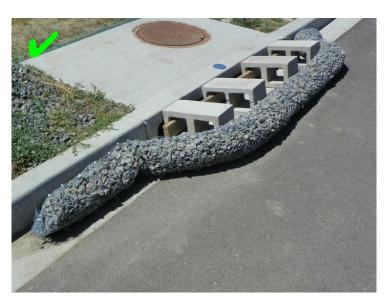
Good example of a sump-style *Inlet Protection* installation with one, long, continuous rock wattle. Note the long interface with the curb facing at each end.
