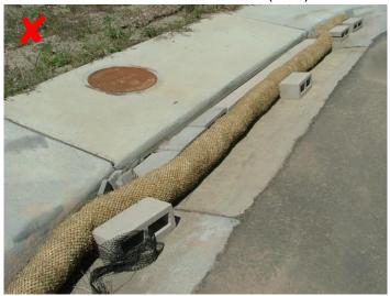
Straw Wattles do not perform well as *Inlet Protection*. They do not filter flows and are prone to by-pass, because their light weight and buoyancy do not allow a good seal with the curb flowline.
