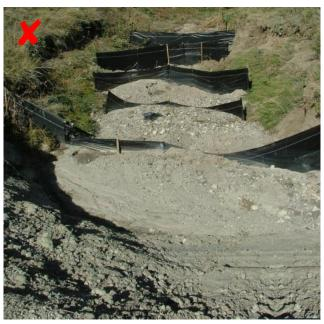
Silt Fence is not designed to work in a concentrated flow. Adding additional rows will not alter that design standard.
