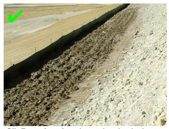
Silt Fence functions best when backed away from the toe of a slope. Note the buffer zone of Surface Roughening here.
