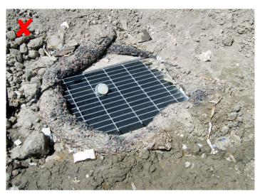
Inlet Protection must be maintained in good operating condition and should not allow sediment to discharge to the box.
