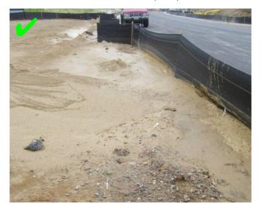
If sited and installed correctly, Silt Fence can perform well as a sediment barrier and to pond storm water.
