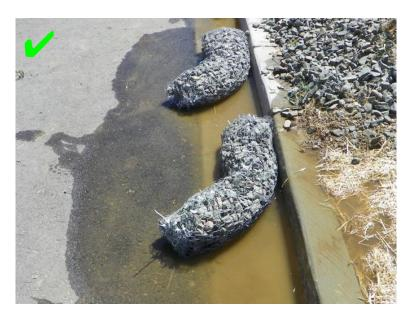
Curb Socks can assist with sediment removal in curb flowlines, prior to discharge to an inlet.
