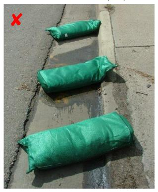
An appropriate style of curb sock must be selected to function as on-grade *Inlet Protection* to prevent by-pass.
