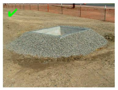
A gravel pack can be installed as a substitute to the wire mesh rock wattles for *Area Inlet Protection*, but may be more difficult to maintain or demolish.
