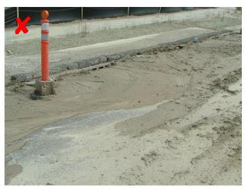
Inlet Protection is not designed to hold back large sediment plumes. The rock wattles are easily clogged, overwhelmed and sediment is discharged to the box.
