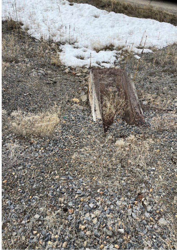
Photograph 8: Top of storm water outlet.
