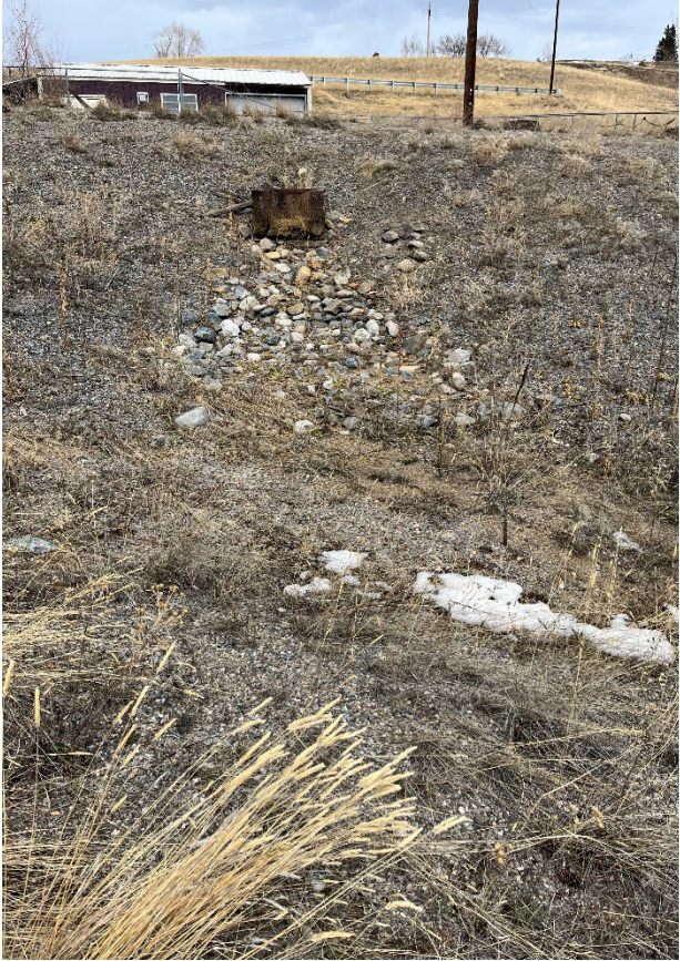
Photograph 7: Storm water outlet looking north.
