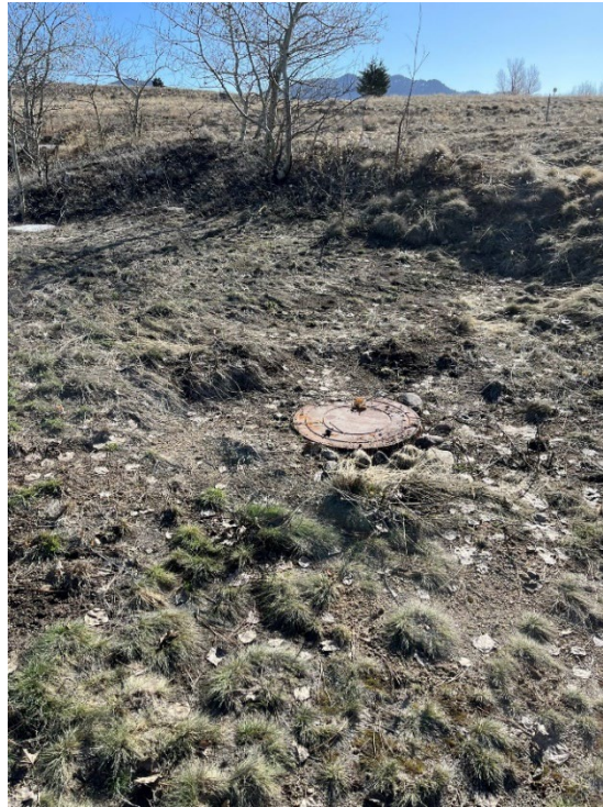
Photograph 4: Manhole located on site.
