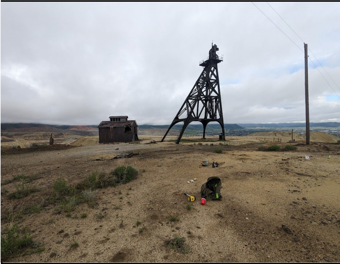
Figure 27: Photo of Bell Headframe
