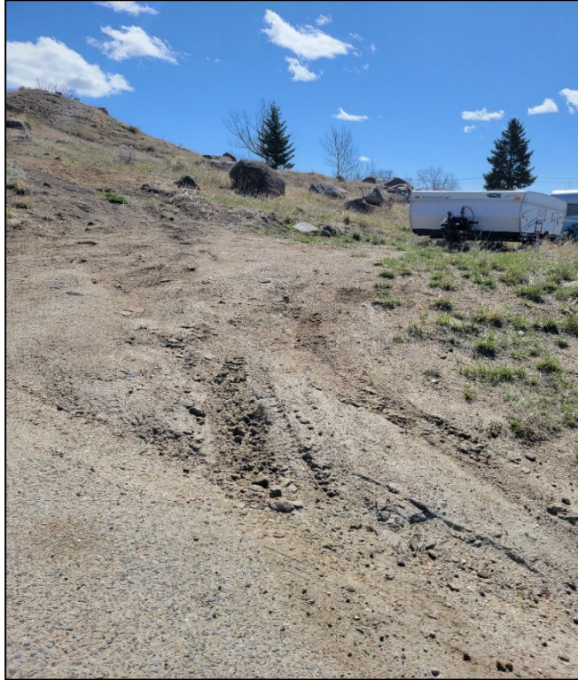
Photograph 4: Sediment Runoff from Site to Road.
