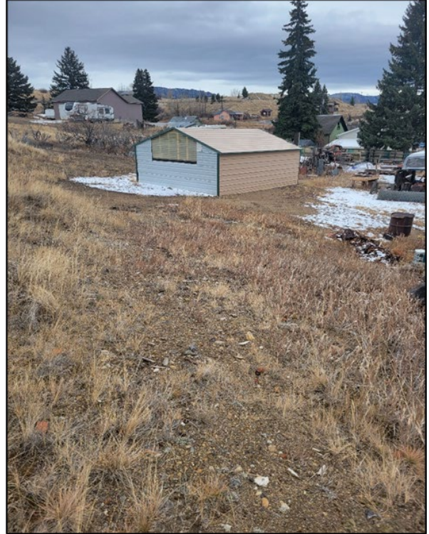
Photograph 4: Barren Area South of Shaft, Active Erosion.
