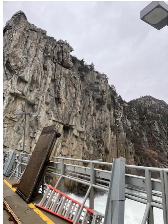
Figure 1: Left abutment rock mass downstream of Madison Dam
