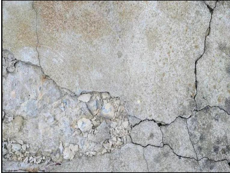
*Figure 8 - Example of Spalling*
