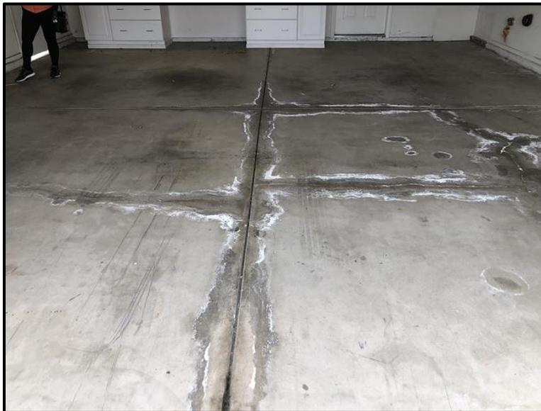
*Figure 6 - Example of Efflorescence Staining*
