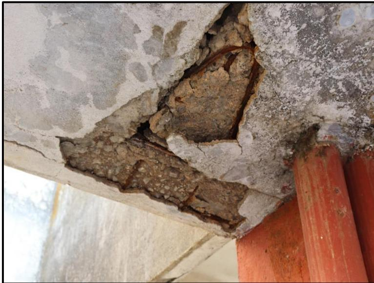
*Figure 7 - Example of Delamination and Exposed Rebar*
