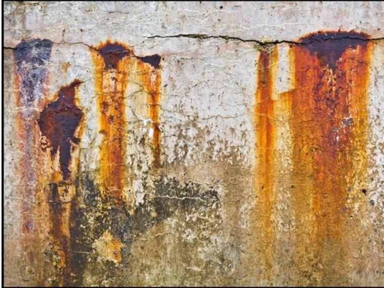
*Figure 5 - Example of Rust Staining*
