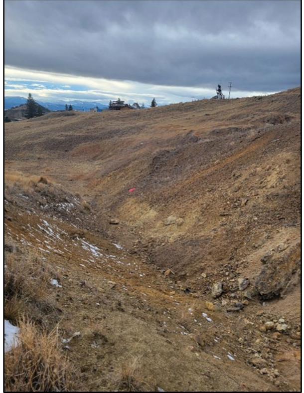
Photograph 3: Steep Eroding Slopes with Iron Staining.
