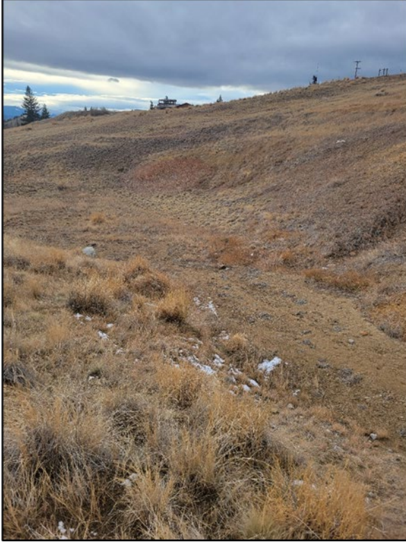
Photograph 3: Area of Soil Deposition from Storm Water Inlet.
