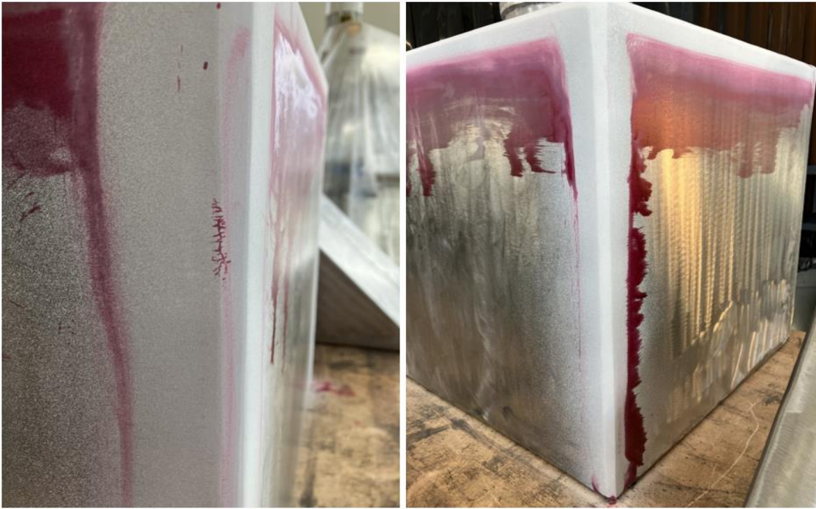
Figure 29: Welded joints after completion of the dye penetrant test depicting an acceptable weld (right) and unacceptable weld with a root crack (left).
