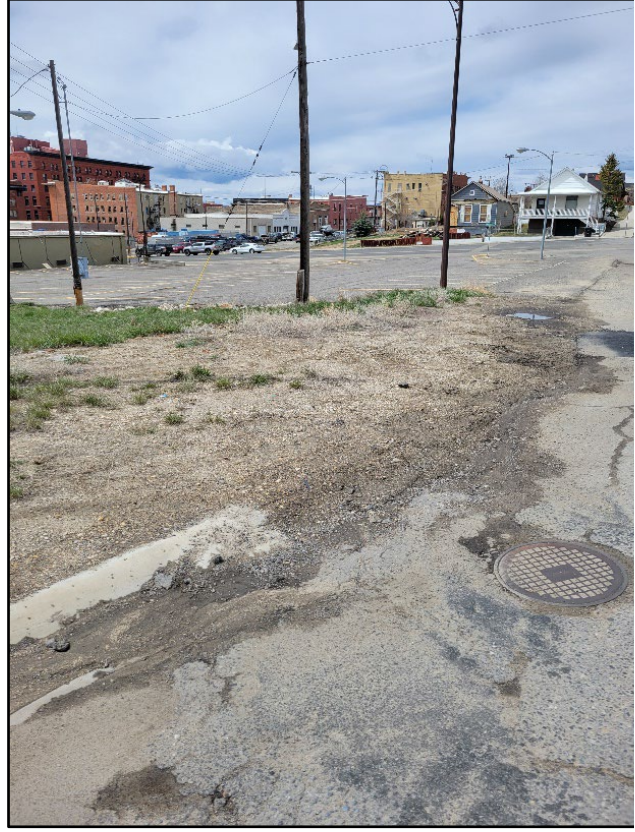
Photograph 2: Sediment Transporting along North Boundary.
