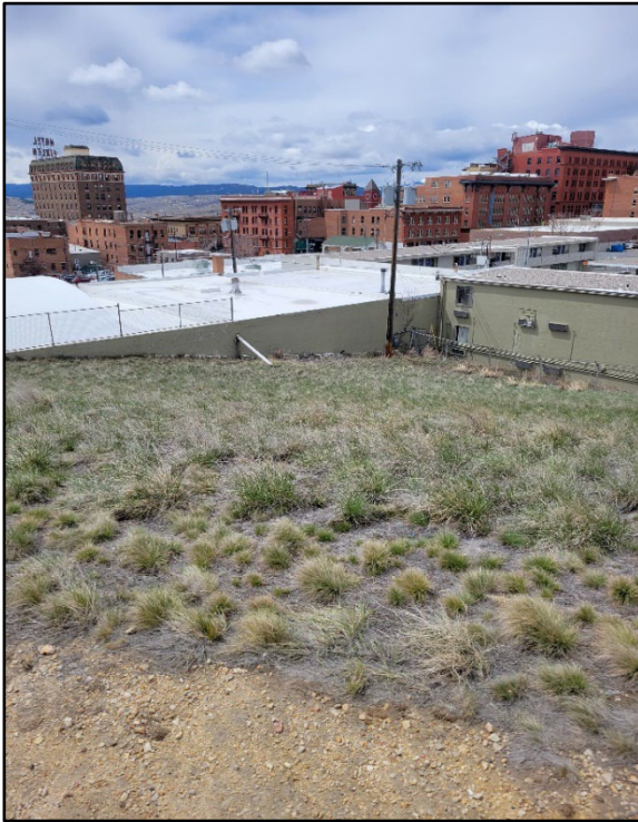
Photograph 3: Storm Water may be Running onto Site from Roof Top.
