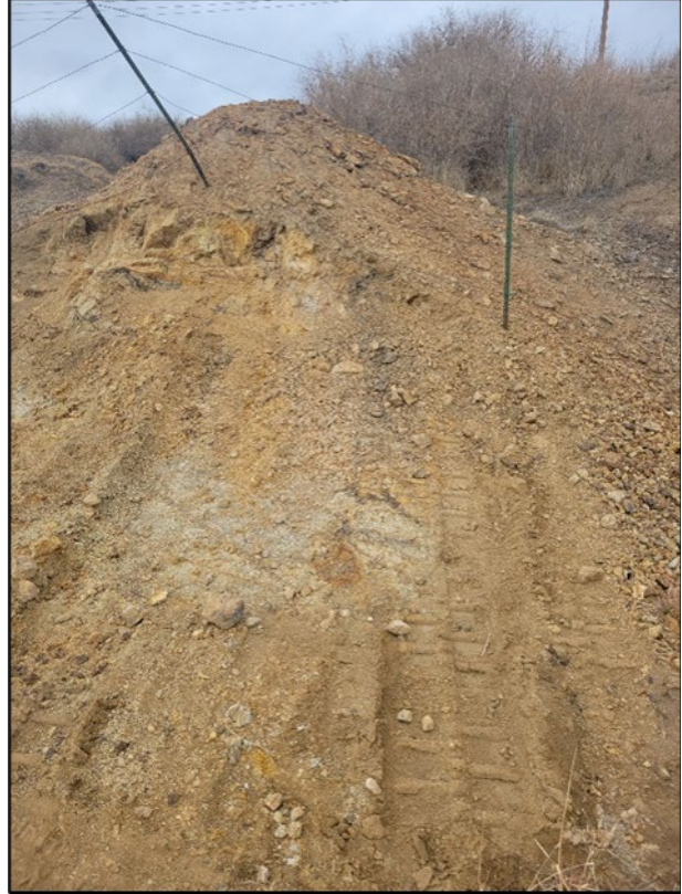
Photograph 9: Barren Area Eroding on South Boundary
