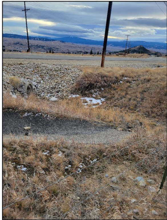
Photograph 2: Storm Water Inlet on Southwest Corner of Site
