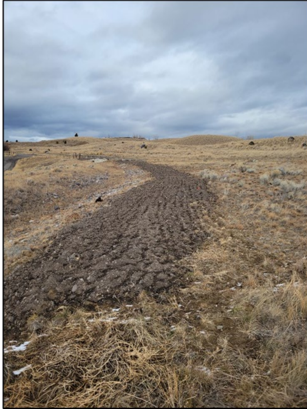
Photograph 5: BSB Remediation Efforts Along Storm Water Channel
