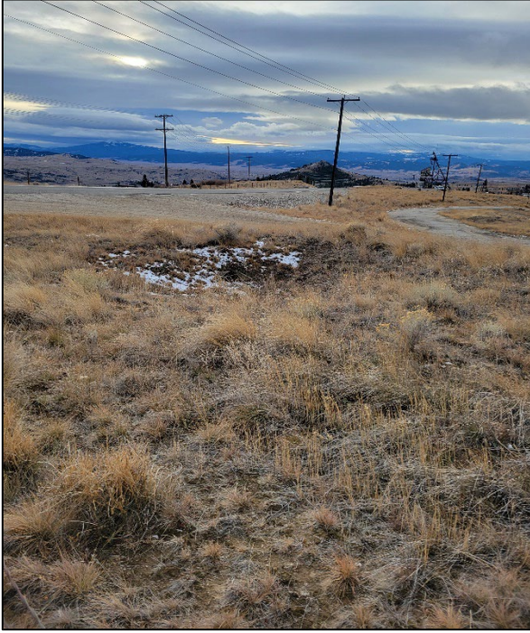
Photograph 3: Asphalt and Concrete Storm Water Features-South
