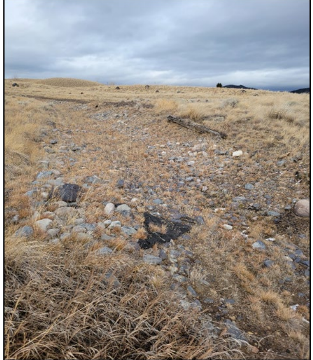
Photograph 4: Rock Lined Storm Channel Through Middle of Site
