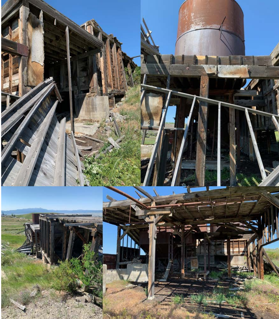
Figure 4. Photos taken on site in 2020 of the various structures on the Marget Ann property.
