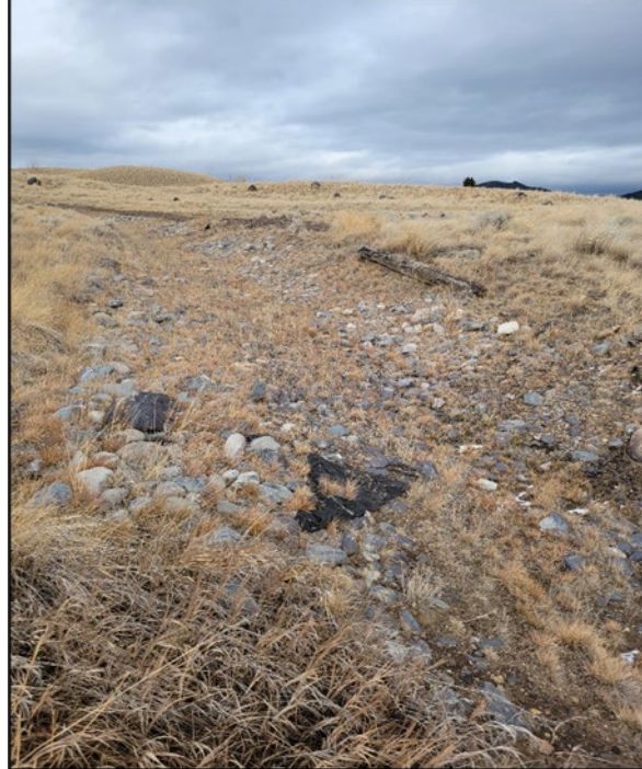
Photograph 4: Rock Lined Storm Channel Through Middle of Site
