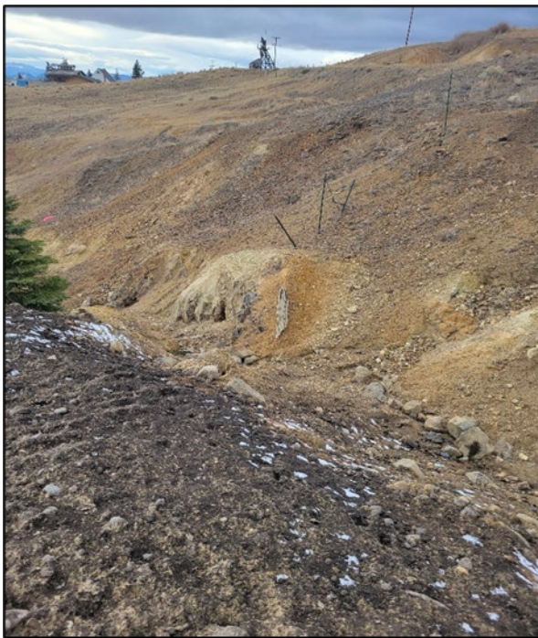
Photograph 4: Edge of BSB Remedial Action and Large Gully.
