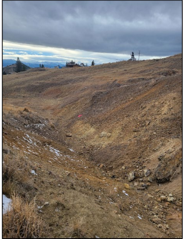
Photograph 3: Steep Eroding Slopes with Iron Staining.
