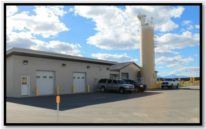
Photograph 1. Operations and CAS Buildings.
