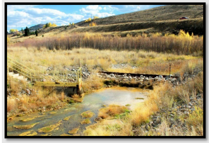
Photograph 3. HCC Sheet Pile Termination Wall.
