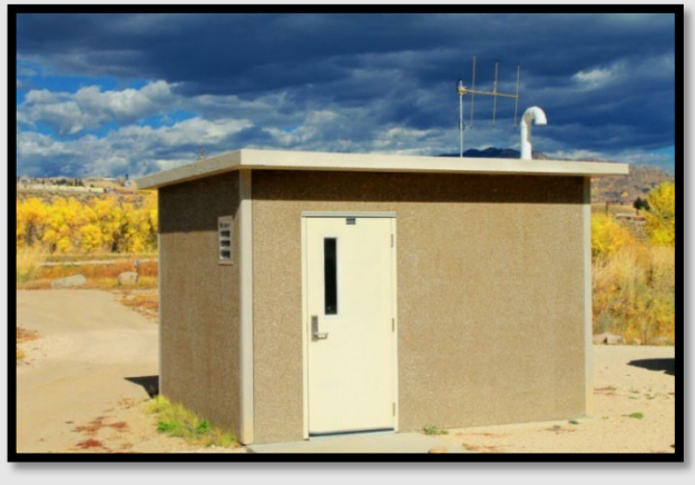
Photograph 2. Automatic Sampling Building.
