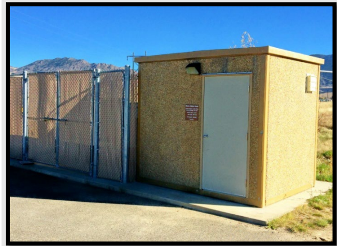
Photograph 5. BPSOU Subdrain Pump Station Control Building
