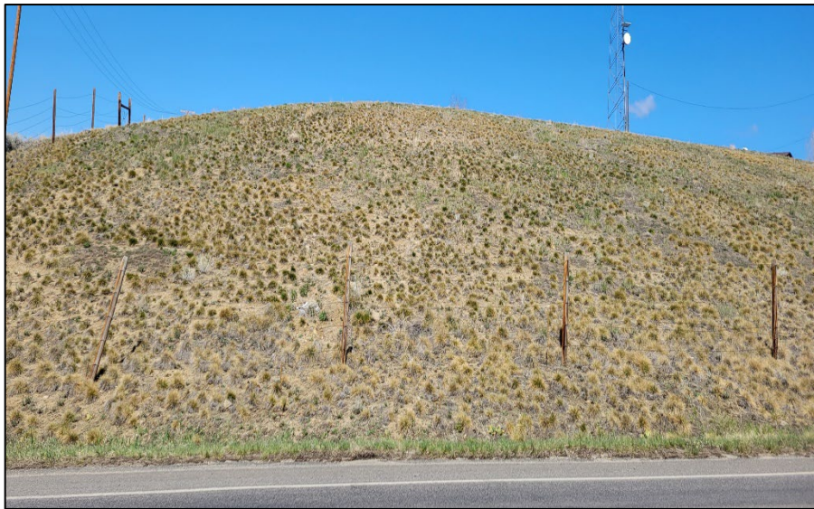
Photograph 6: East Facing Slope has Grass Establishment, Very Patchy.
