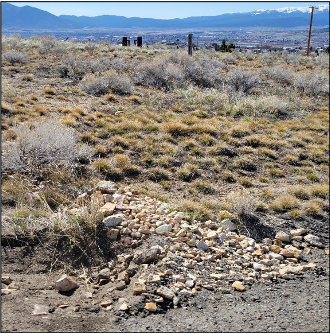
Photograph 5: Temporary Best Management Practices along West Boundary. Evidence of Sediment Migration.
