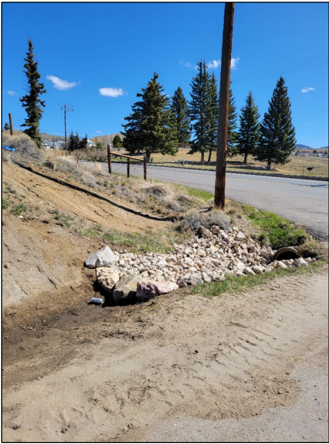
Photograph 4: Sediment Control on Southeast Corner of Site Capturing Sediment Migration.
