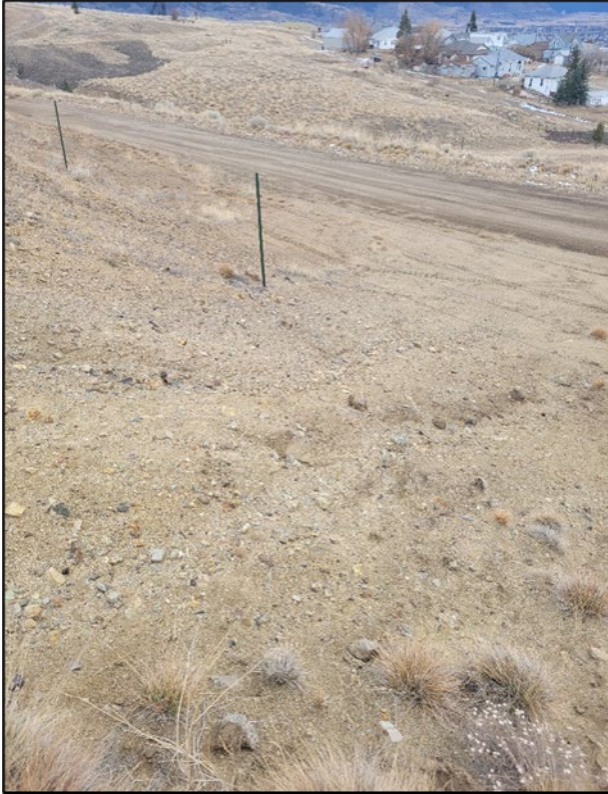
Photograph 1: Erosion Rills Active on South Slope
