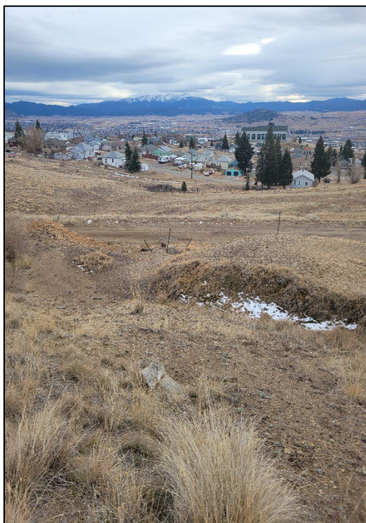
Photograph 5: Gully Developing Near Possible Mine Dump (South Boundary)
