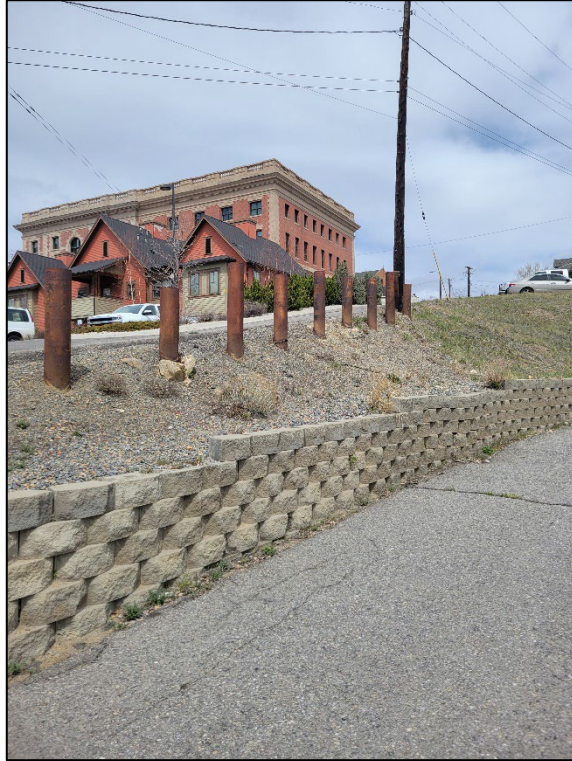
Photograph 2: Butte-Silver Bow Noted a Collapsed Steam Line.
