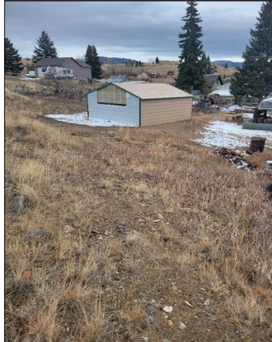
Photograph 4: Barren Area South of Shaft, Active Erosion.
