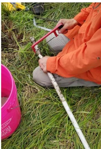
**Figure 7: Hand cutting well screen slots with a hacksaw**
