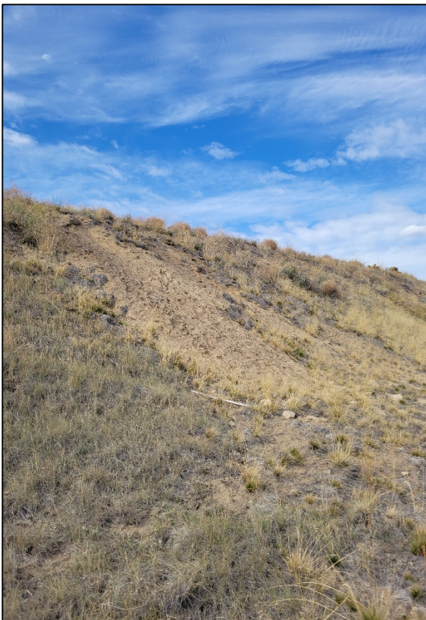
Photograph 1. Possible Mining Waste Erosion
