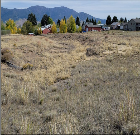
Photograph 5. South Storm Water Sediment Ditch
