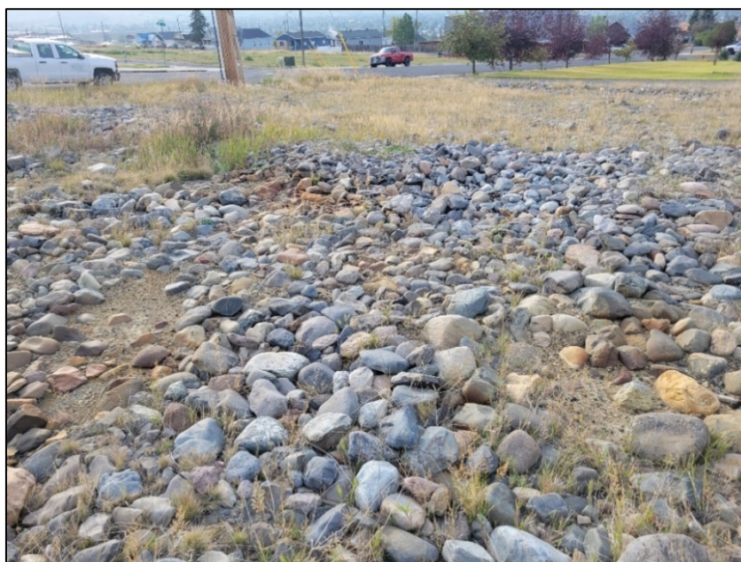
Photograph 1. Possible Mining Waste Leaching Through Rock Cap
