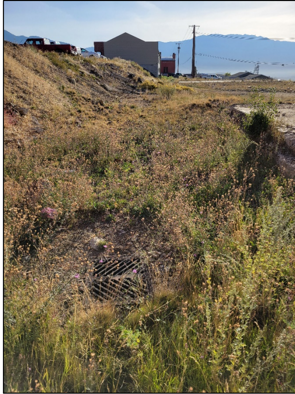
Photograph 3. Manhole AB-M-2201 Located North of Concrete Foundation
