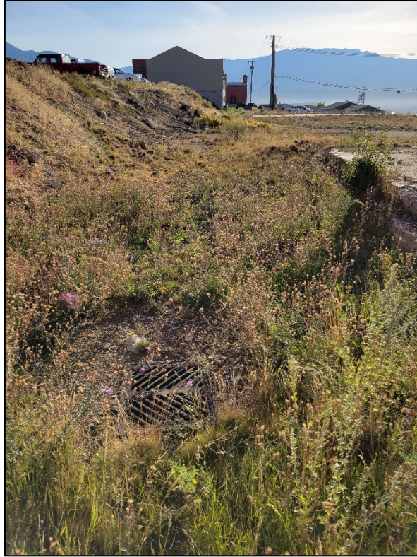
Photograph 3. Manhole AB-M-2201 Located North of Concrete Foundation
