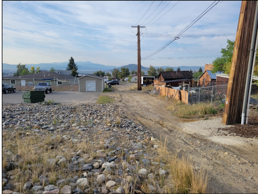
Photograph 2. Storm Water Flows Causing Rills that Transport Material to the South End of the Alleyway.
