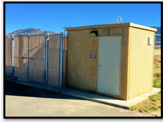
Photograph 5. BPSOU Subdrain Pump Station Control Building
