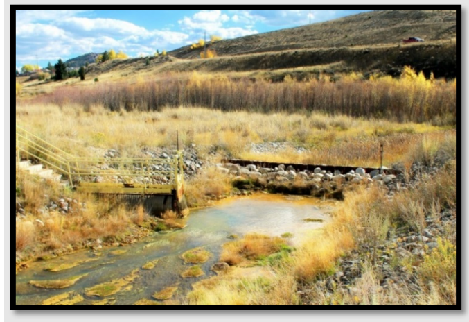
Photograph 3. HCC Sheet Pile Termination Wall.
