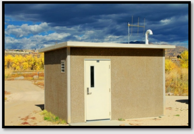
Photograph 2. Automatic Sampling Building.
