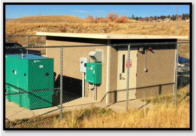
Photograph 4. West Camp Pump Station.
