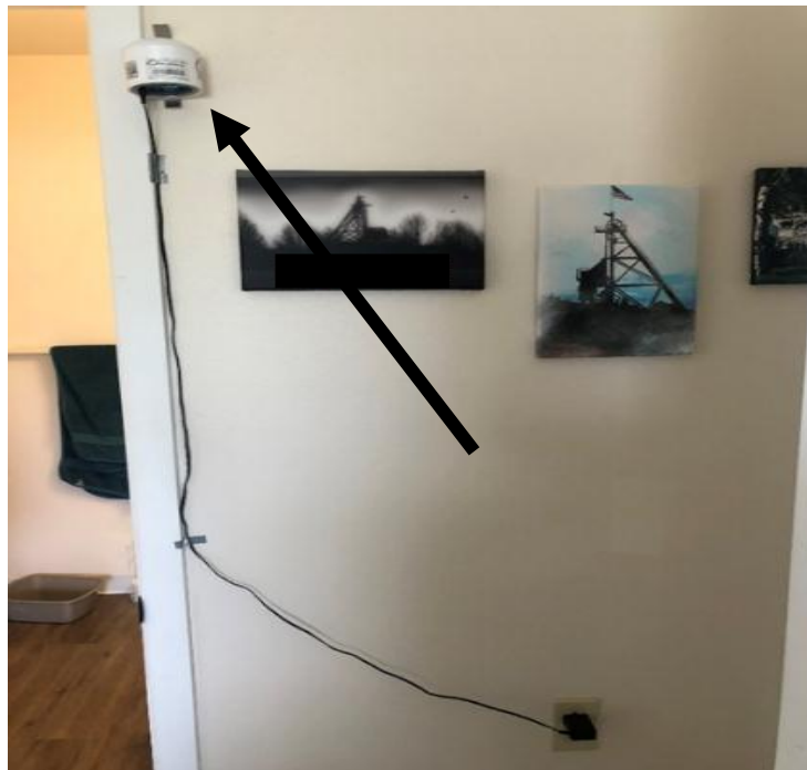
Figure 5. PurpleAir Setup @ Facility 2
