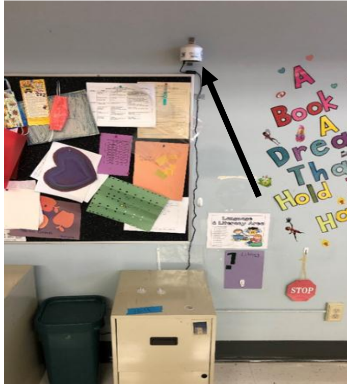
Figure 8. PurpleAir Setup @ Facility 3
