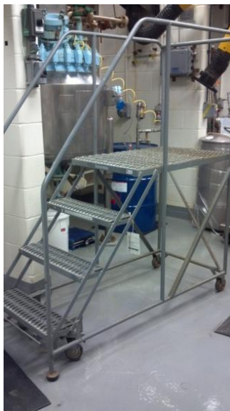
Figure 2: View of the elevated platform with reactor in the background
