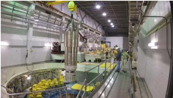
64,000-pound inner reflector plug being lowered into position at SNS
