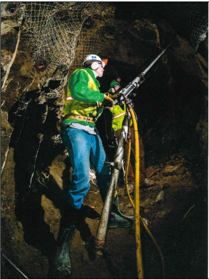
Figure 20. Student using a jackleg drill.
