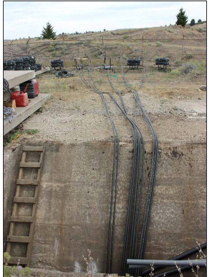
Figure 10. Poly lines being lowered down ventilation shaft.
