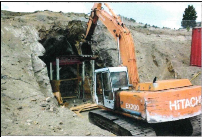
Figure 4. Constructing the Portal.
