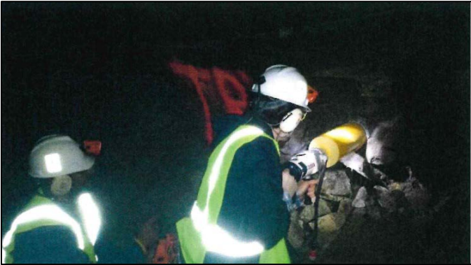
Figure 16. Drilling 6 inch hole in pillar.
