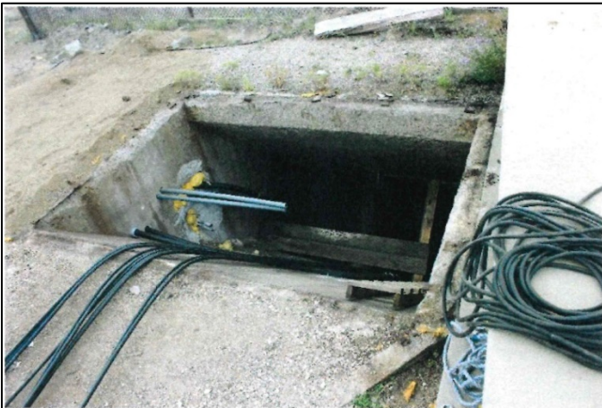
Figure 12. Looking down ventilation shaft.
