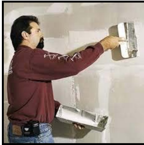
Figure 3 – Example of Applying Wet Joint Compound
