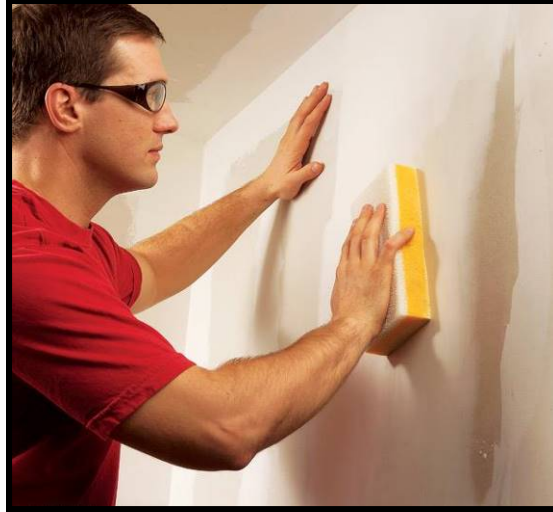
Figure. 5 – Example of Wet Sanding
