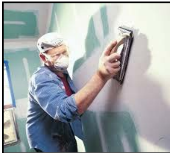
Figure. 4 – Example of Dry Sanding
