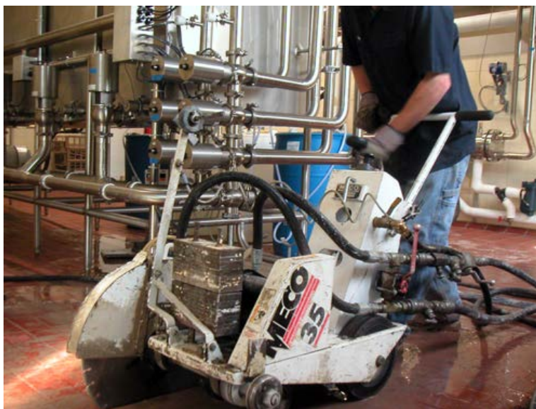
Figure. 2 – Example of Concrete Saw Cutting in a Basement
