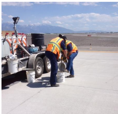
Figure 21 Mixing Epoxy
