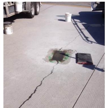
Figure 22 Curing Epoxy
