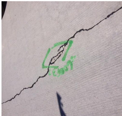
Figure 17 Concrete Crack
