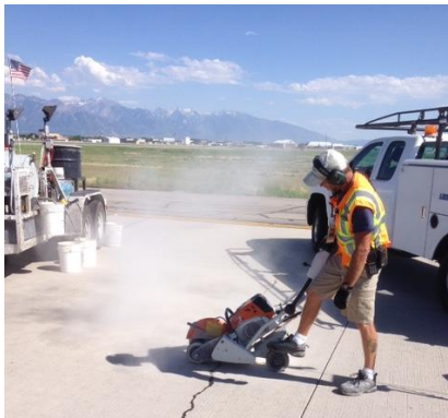
Figure 18 Concrete Cutting
