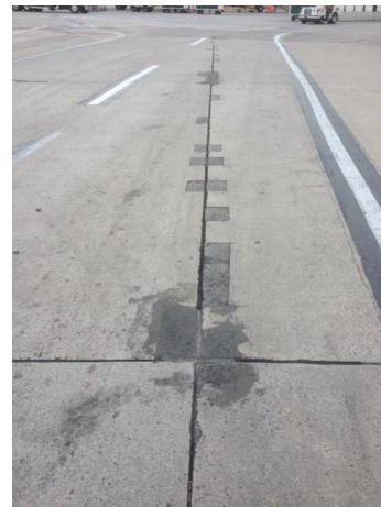
Figure 10 Airfield Concrete Repair
