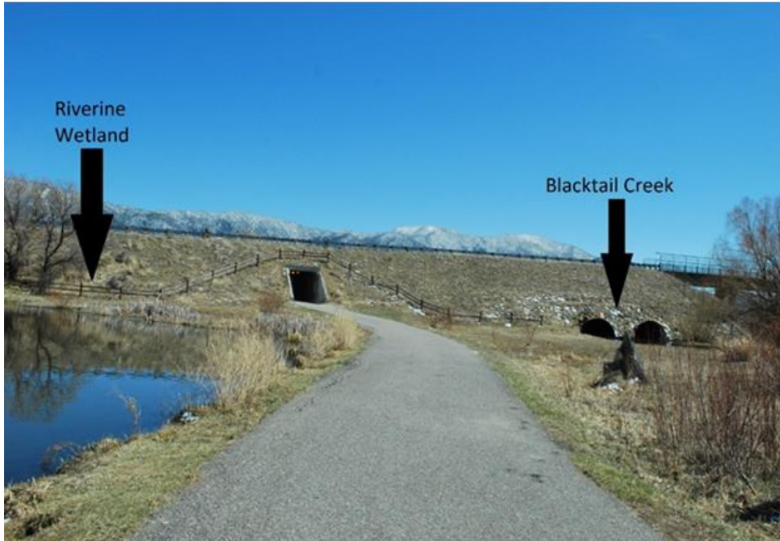
Figure 3: Walking Trail/Levee (facing East)
